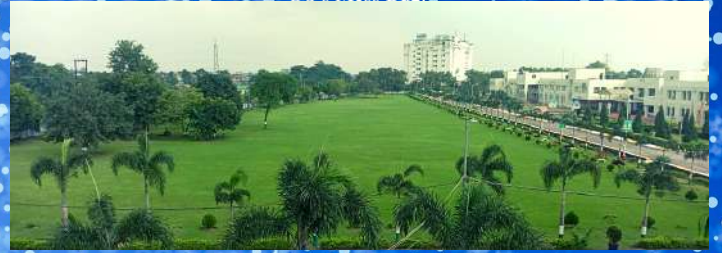
Admin. Block, Quarter Guard & Store Block
